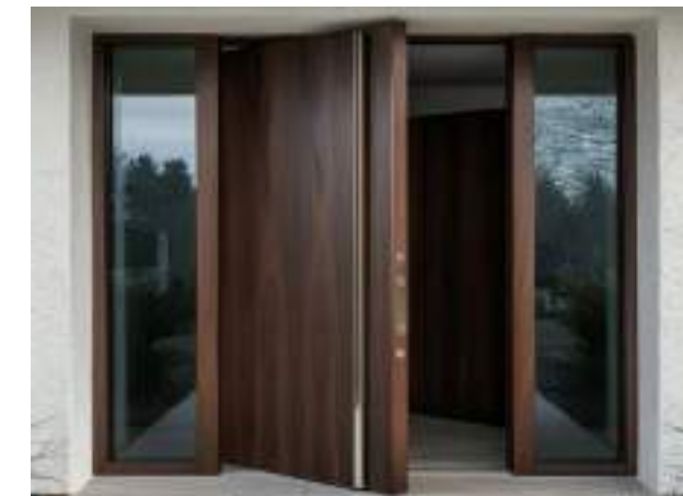
Ground Floor Entrance door – Hardwood timber
