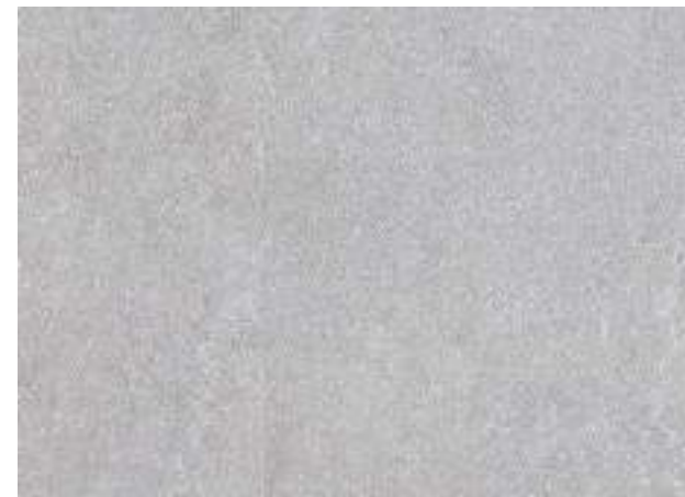
Ground Floor Exterior Wall Finish – Plaster & Paint
